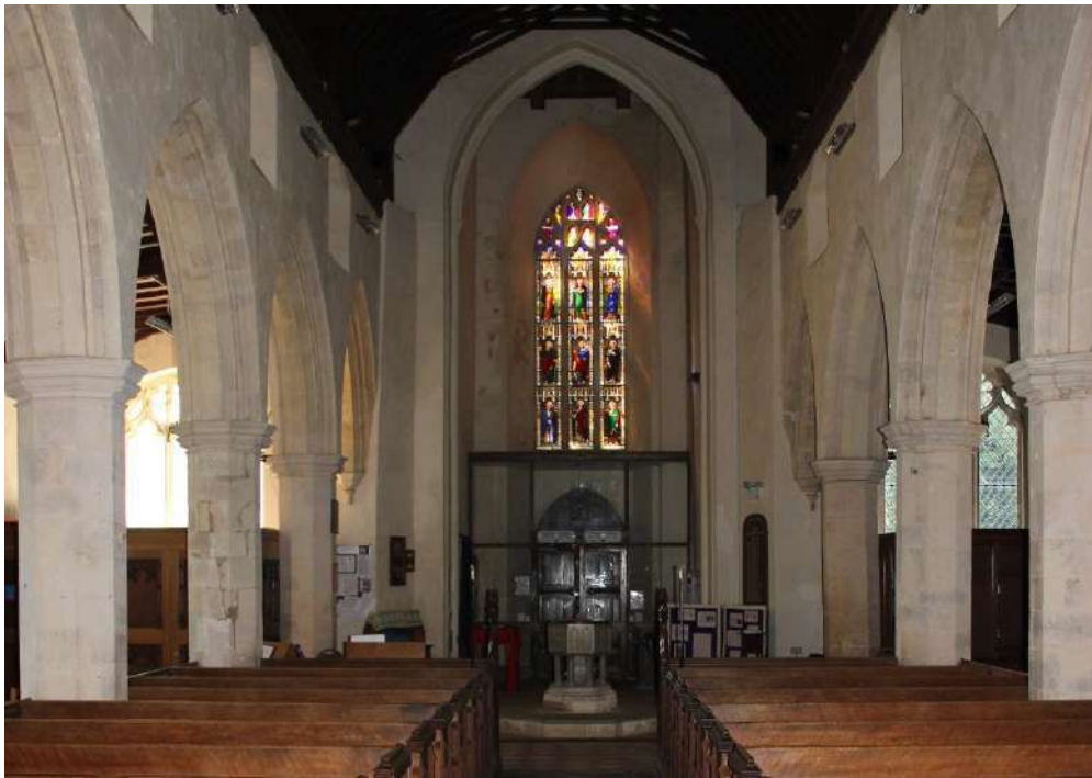
Fig 5. Tower of All Saints Church Filby from the Nave
